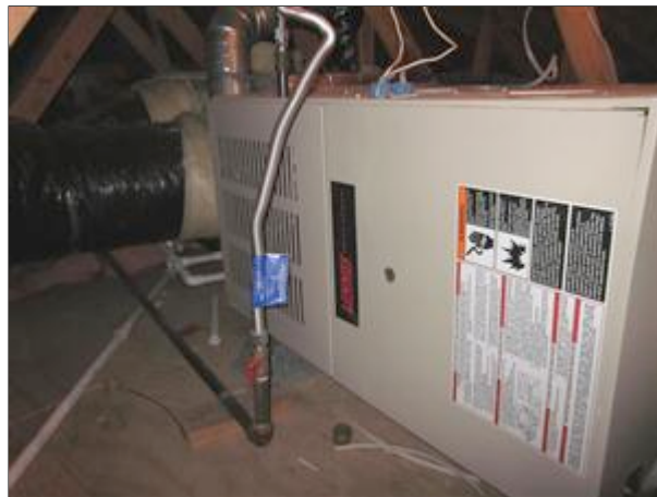
7.0 Picture 1 attic view
