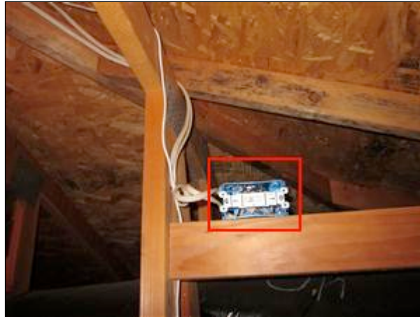
4.5 Picture 1 attic view
